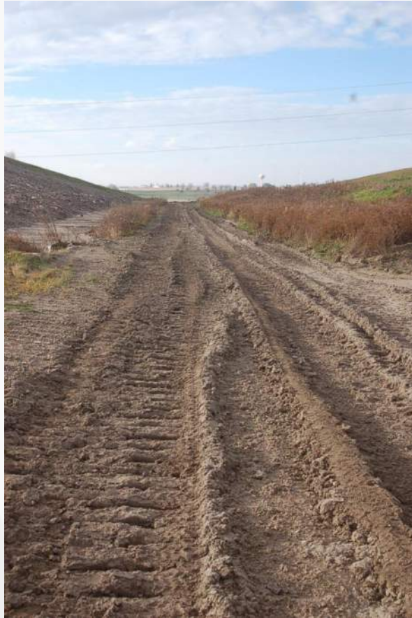
Photo 25 - Cell 2 East Perim Road/Toe of LF Face
