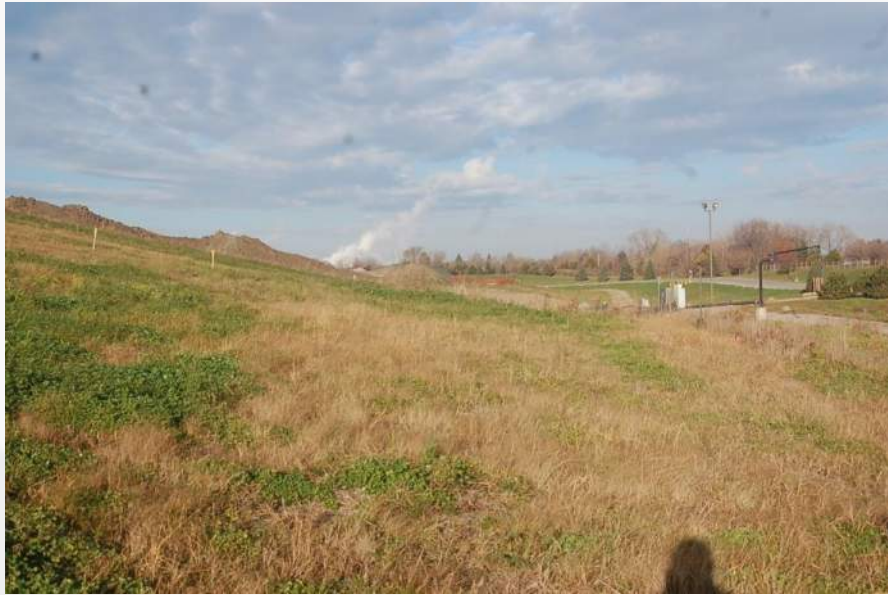
Photo 1 - Cell 3 North Landfill Face
