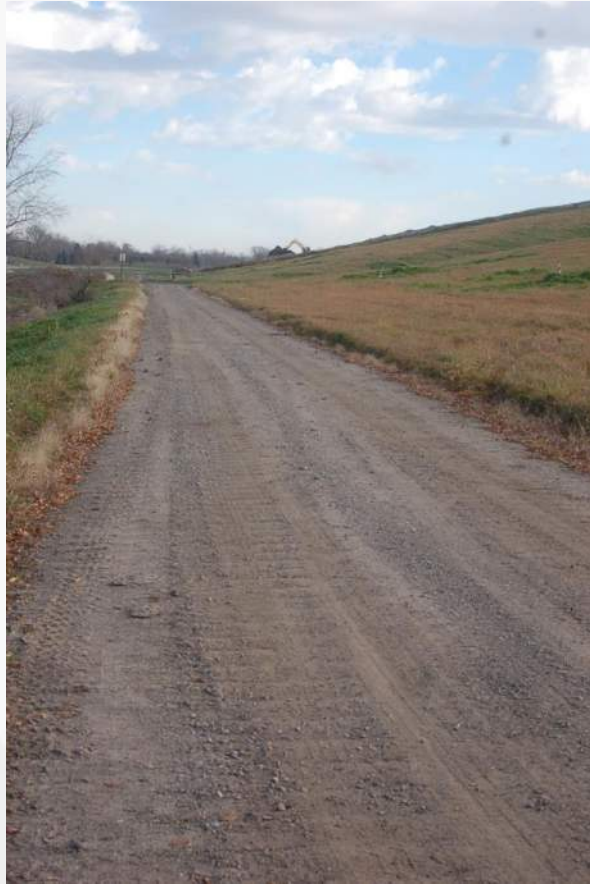
Photo 59 - Cell 2 West Perim Road/Toe of LF Face
