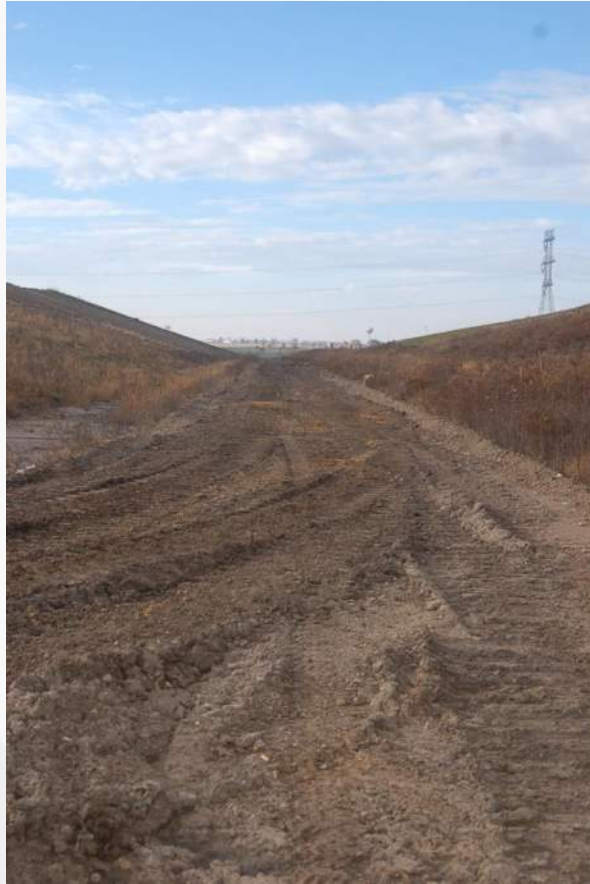
Photo 21 - Cell 3 East Perim Road/Toe of LF Face
