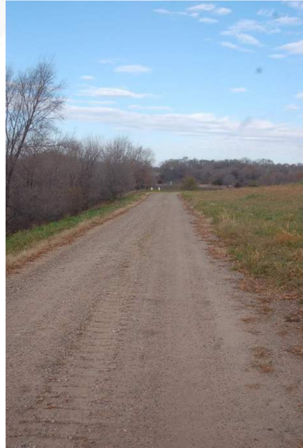
Photo 52 - Cell 2 South Perim Road/Toe of LF Face
