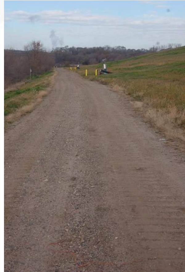
Photo 46 - Cell 2 South Perim Road/Toe of LF Face
