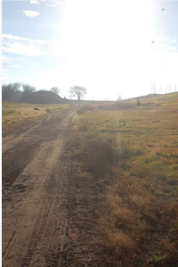
Photo 3 - Cell 3 North Perim Road/Toe of LF Face
