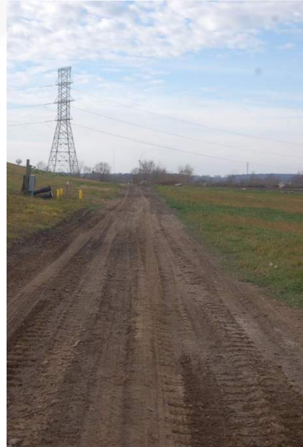
Photo 74 - Cell 1 West Perim Road/Toe of LF Face
