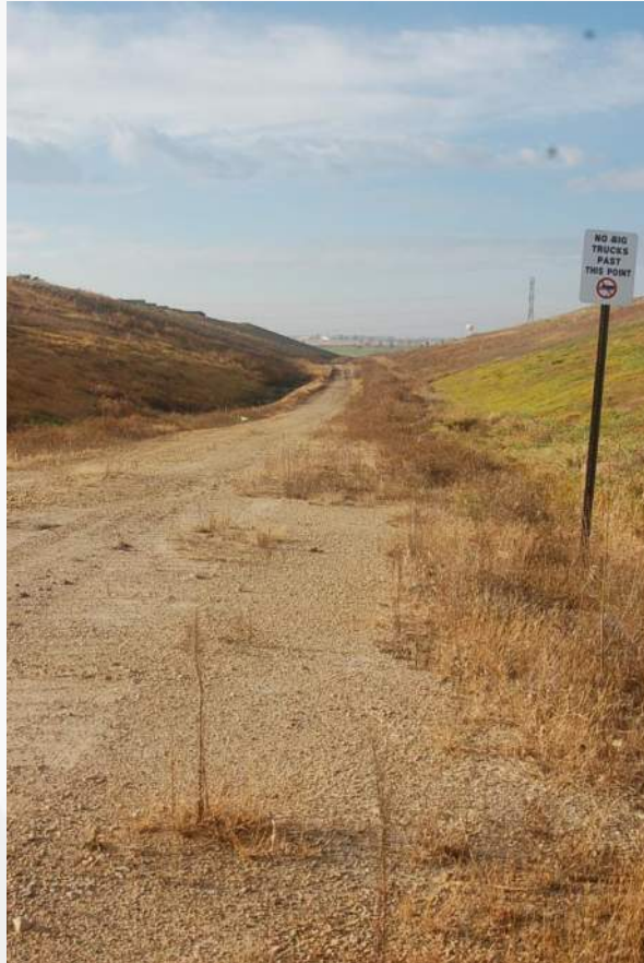
Photo 11 - Cell 3 East Perim Road/Toe of LF Face
