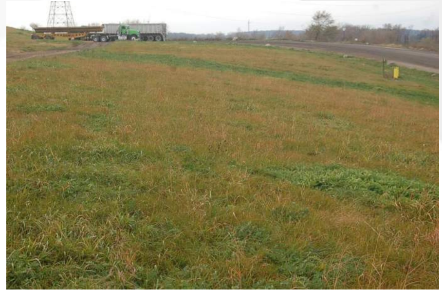
Photo 76 - Cell 1 West Perimeter Berm
