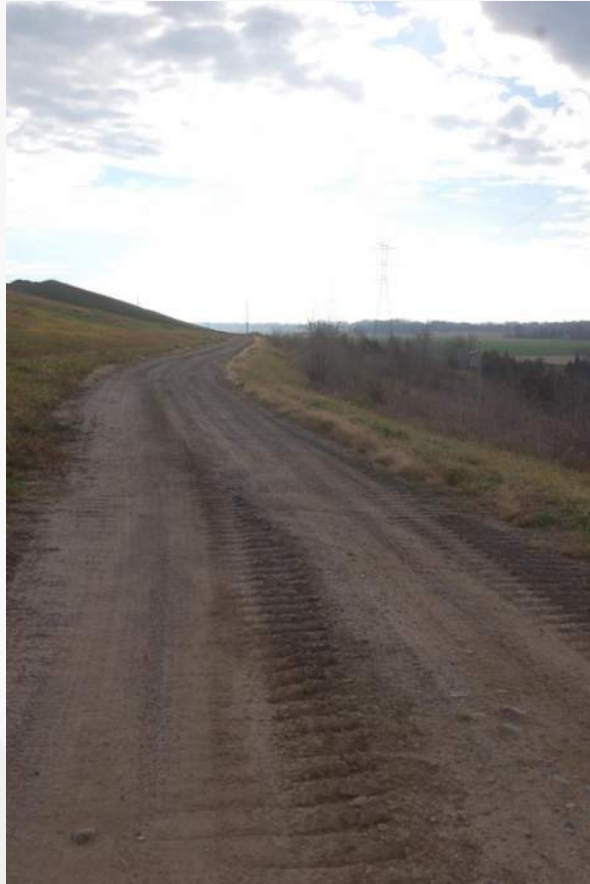
Photo 45 - Cell 2 South Perim Road/Toe of LF Face
