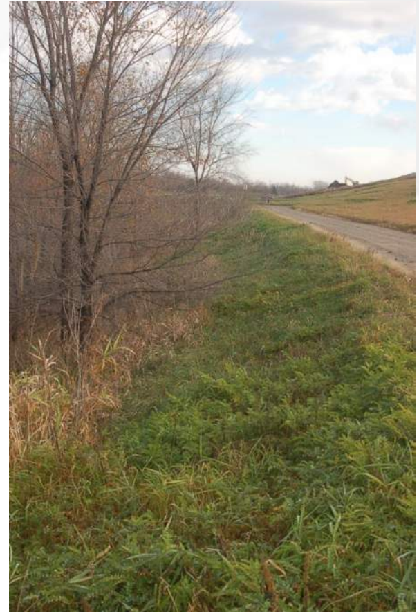
Photo 60 - Cell 2 West Perimeter Berm
