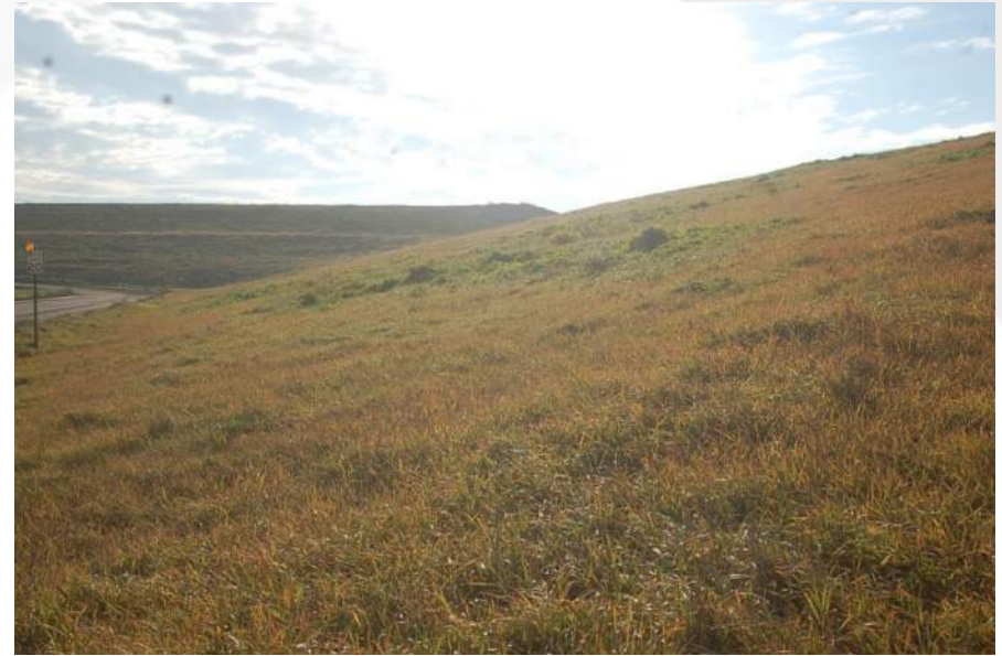
Photo 64 - Cell 2 North Landfill Face
