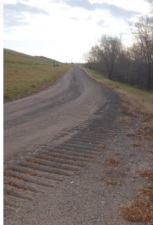
Photo 56 - Cell 2 South Perim Road/Toe of LF Face
