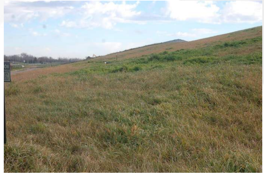
Photo 58 - Cell 2 West Landfill Face
