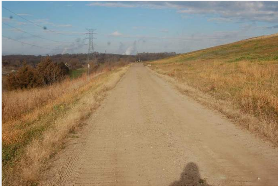
Photo 35 - Cell 2 South Perim Road/Toe of LF Face
