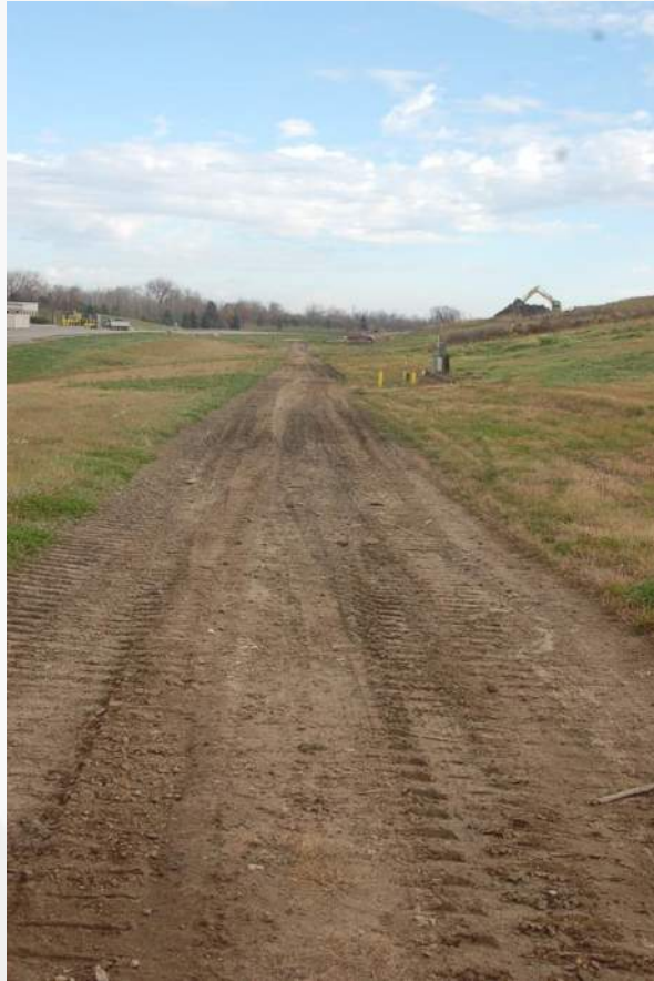
Photo 73 - Cell 1 West Landfill Face
