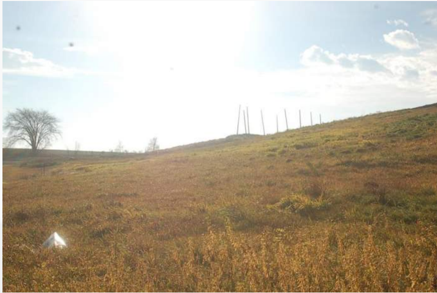
Photo 5 - Cell 3 North Landfill Face
