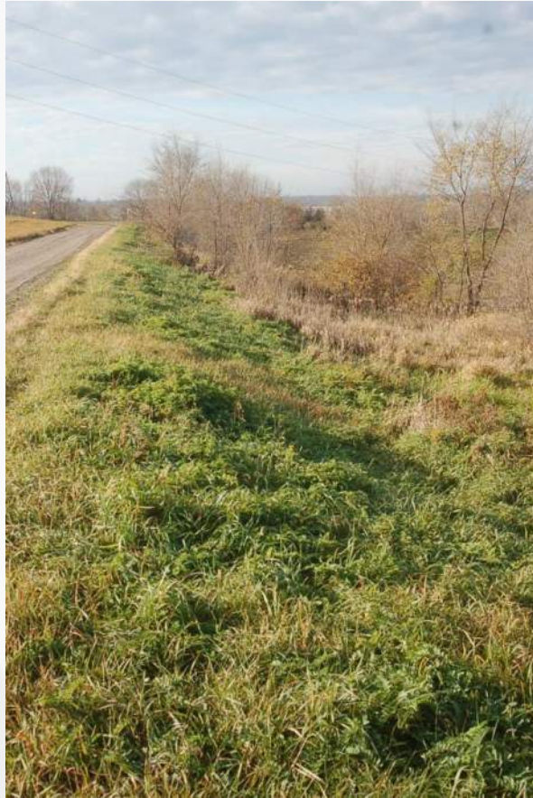
Photo 63 - Cell 2 West Perimeter Berm
