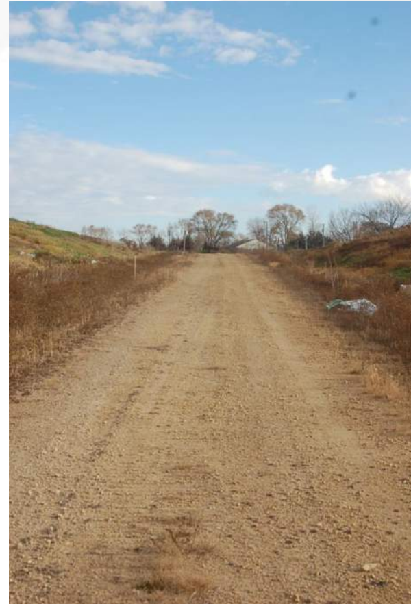
Photo 12 - Cell 3 East Perim Road/Toe of LF Face
