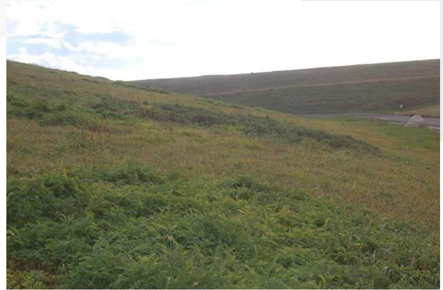
Photo 70 - Cell 3 West Landfill Face
