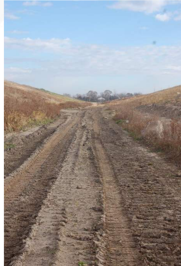
Photo 28 - Cell 2 East Perim Road/Toe of LF Face
