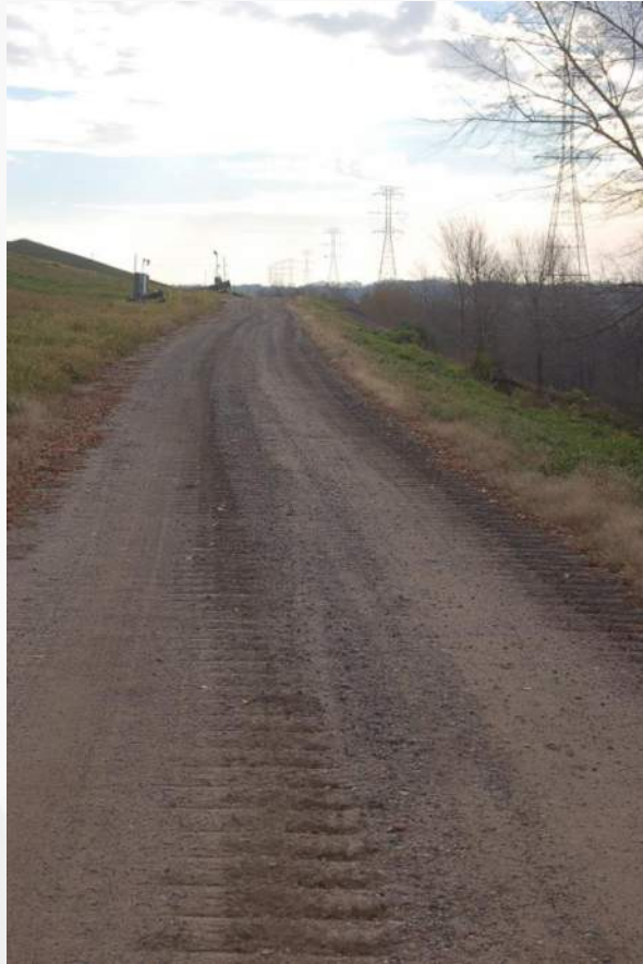
Photo 51 - Cell 2 South Perim Road/Toe of LF Face
