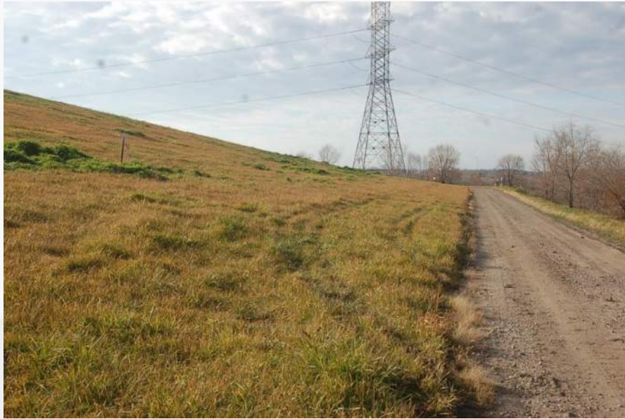
Photo 61 - Cell 2 West Landfill Face
