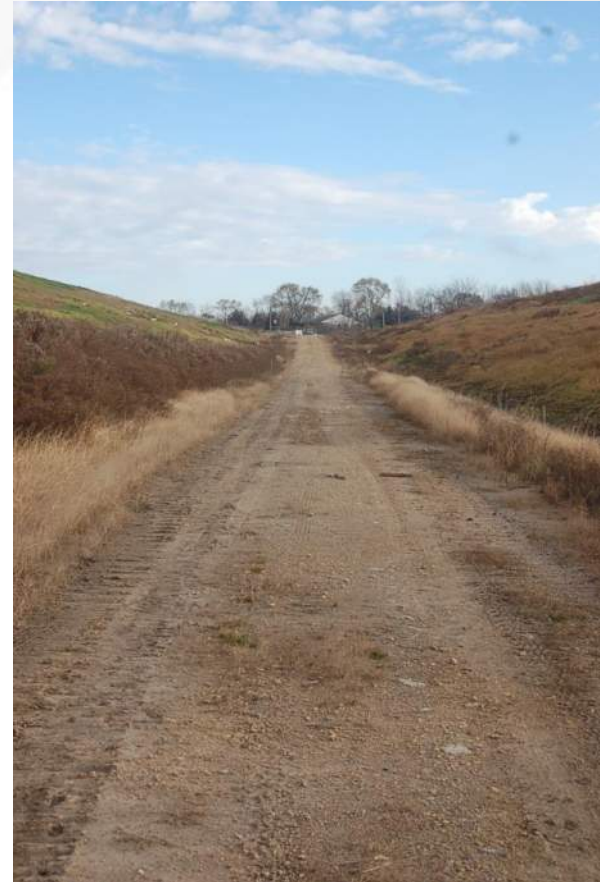
Photo 16 - Cell 3 East Perim Road/Toe of LF Face
