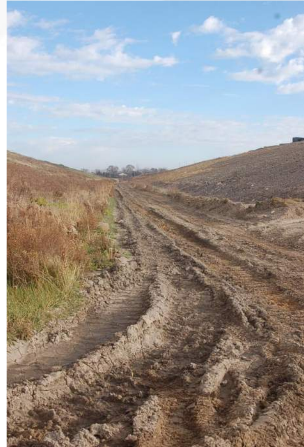
Photo 32 - Cell 2 East Perim Road/Toe of LF Face
