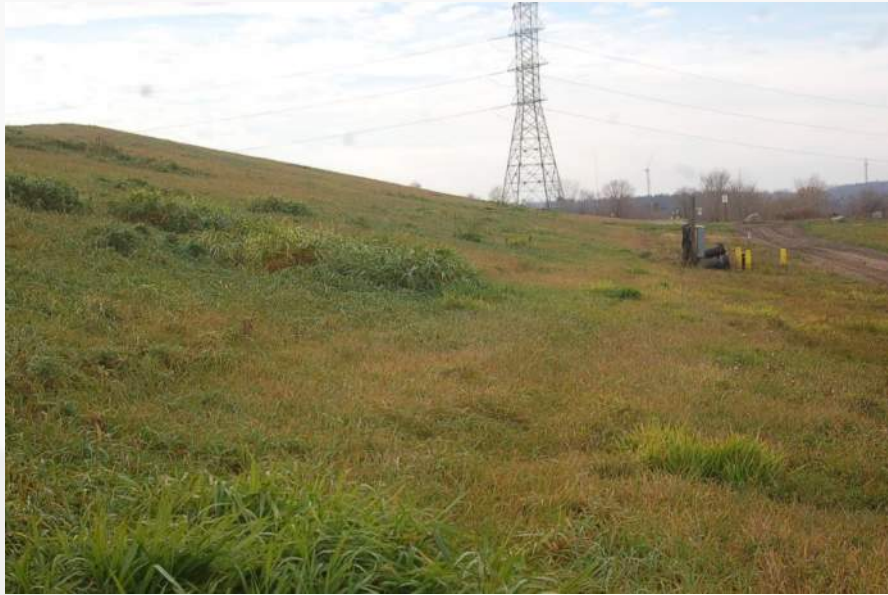
Photo 75 - Cell 1 West Landfill Face
