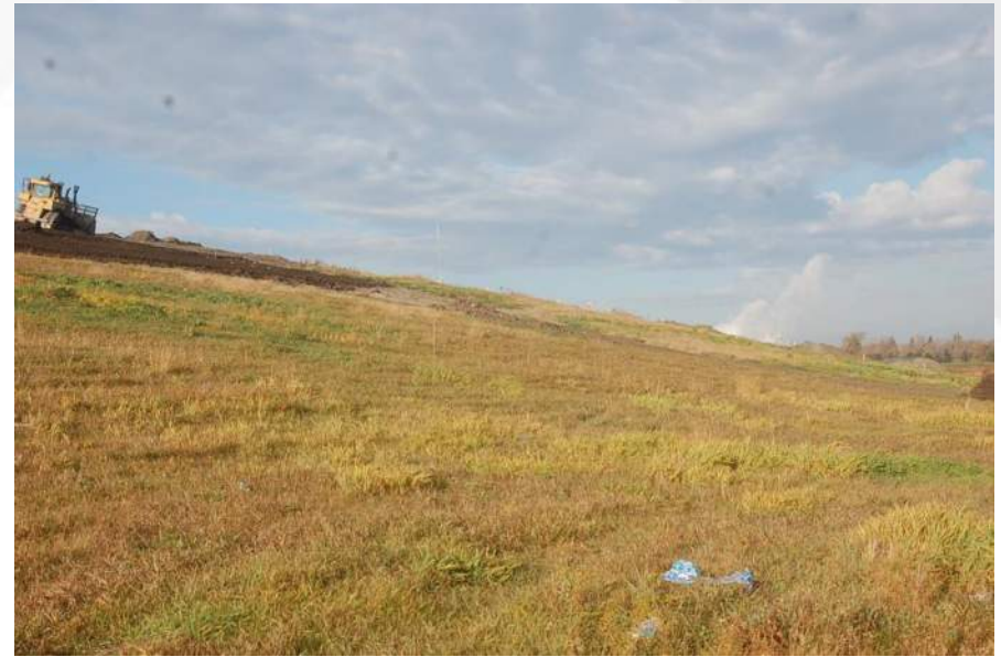
Photo 4 - Cell 3 North Landfill Face
