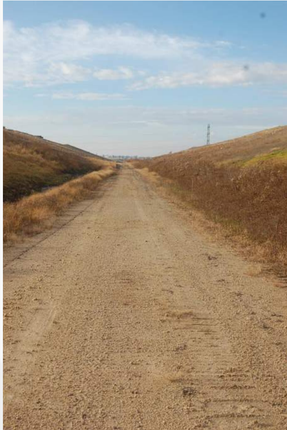
Photo 13 - Cell 3 East Perim Road/Toe of LF Face
