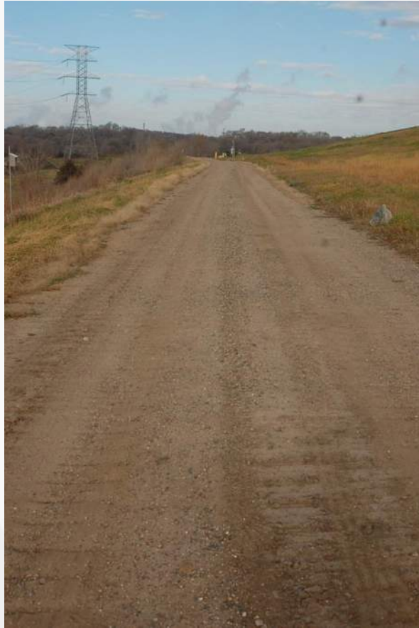
Photo 39 - Cell 2 South Perim Road/Toe of LF Face
