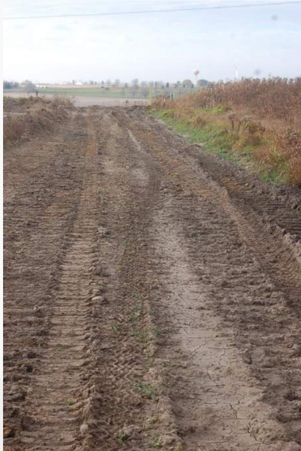
Photo 29 - Cell 2 East Perim Road/Toe of LF Face
