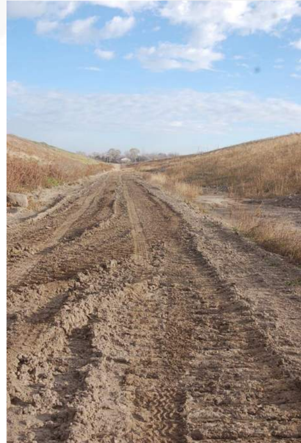
Photo 24 - Cell 3 East Perim Road/Toe of LF Face
