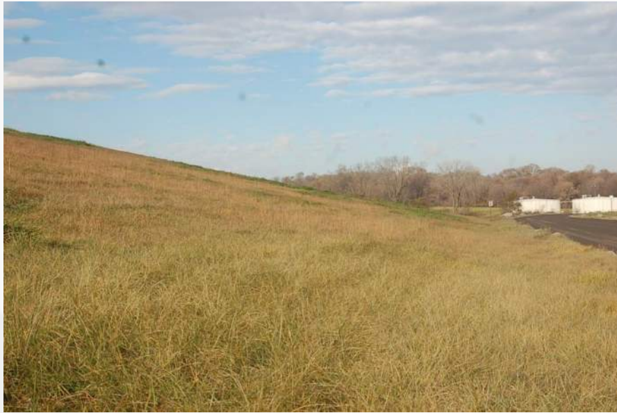
Photo 65 - Cell 2 North Landfill Face
