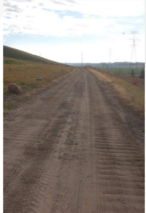
Photo 40 - Cell 2 South Perim Road/Toe of LF Face
